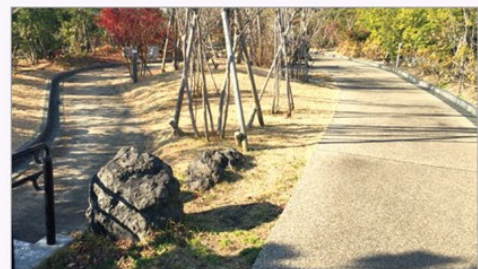
Compared to concrete and asphalt, soil pavement is more porous, allowing water to penetrate easily, which helps to control temperature rise. It doesn't become muddy like plain soil, making maintenance easier.
